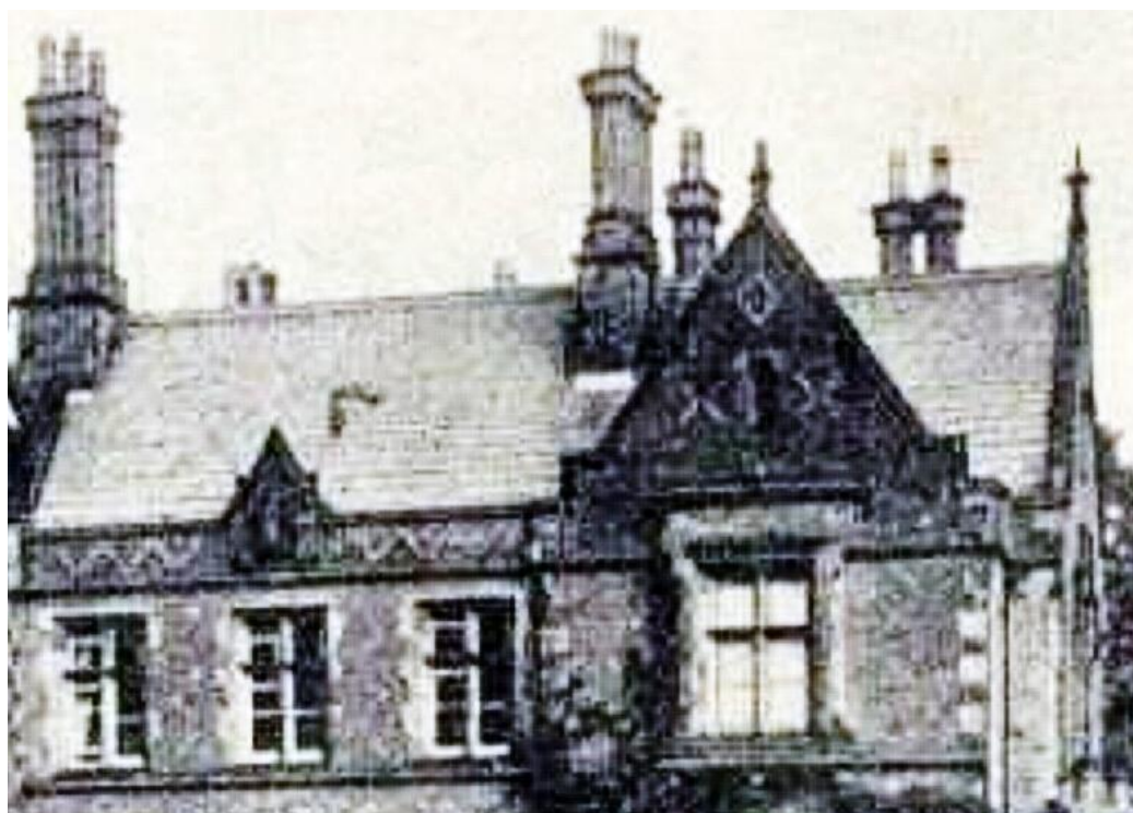
Figure 4: Detail of Woodlands showing the decorative brickwork.
